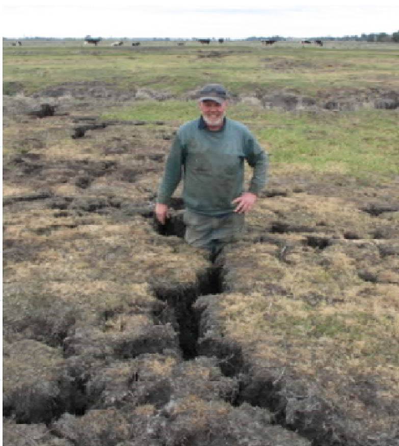
Figure 3. Floodplain Cracking, Heaving & Subsidence (LMIA Irrigation Bay Pompoota). Photo courtesy of the Department for Water.
