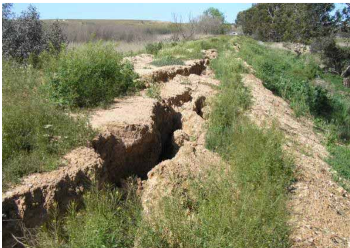
Bank collapse at Neeta. Photo courtesy of the Department for Water.
