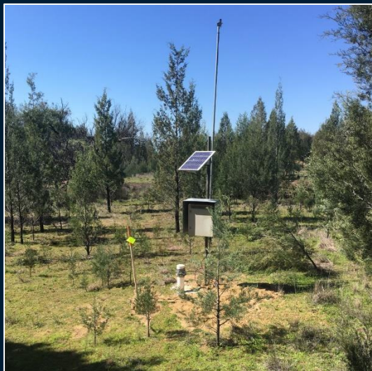
Tiltmeter measurement site, Bowen Basin, Australia
