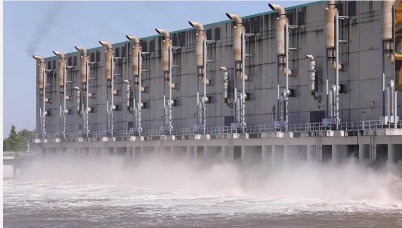
West Closure Sector Gate, New Orleans, USA
