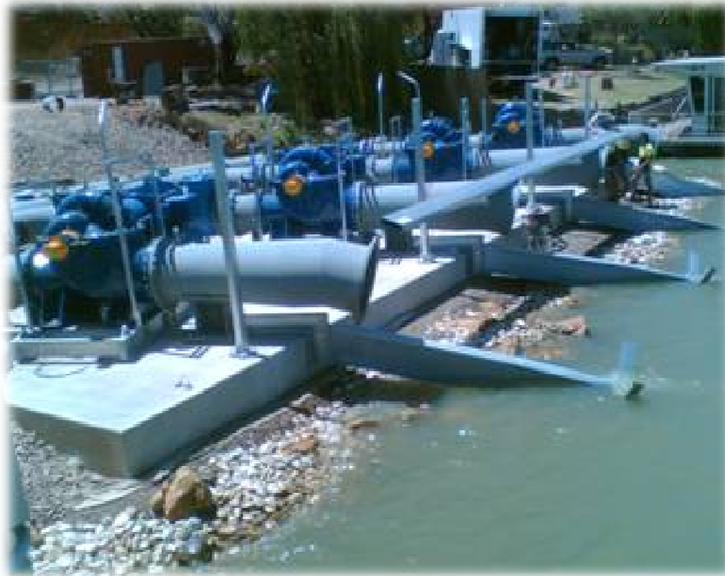
Low-lift pumps being installed at Mannum
