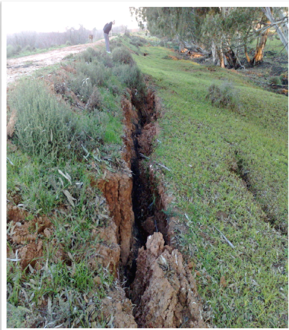
Levee Bank Damage
