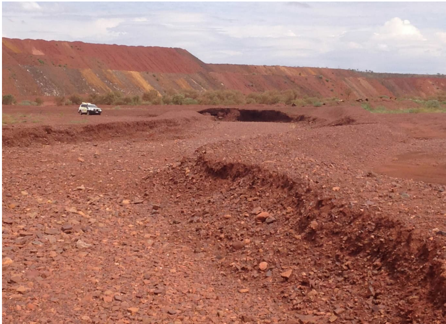
Compaction unsuccessful due to low fines content
