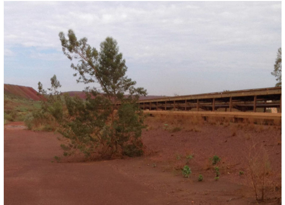
Embankment in Excellent Condition (15 years old)
