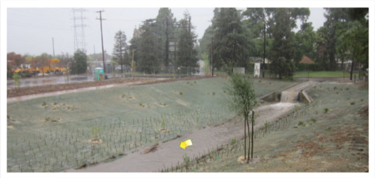
Atwater Park 2011. Daylighted Storm Drain
