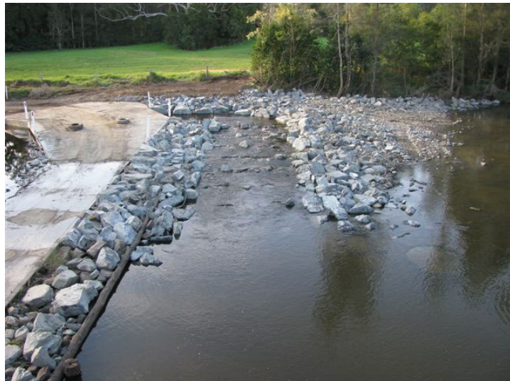
Bypass rock ramp fishway
