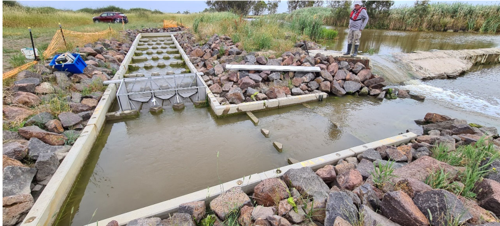
Cone Fishway to eliminate drops
