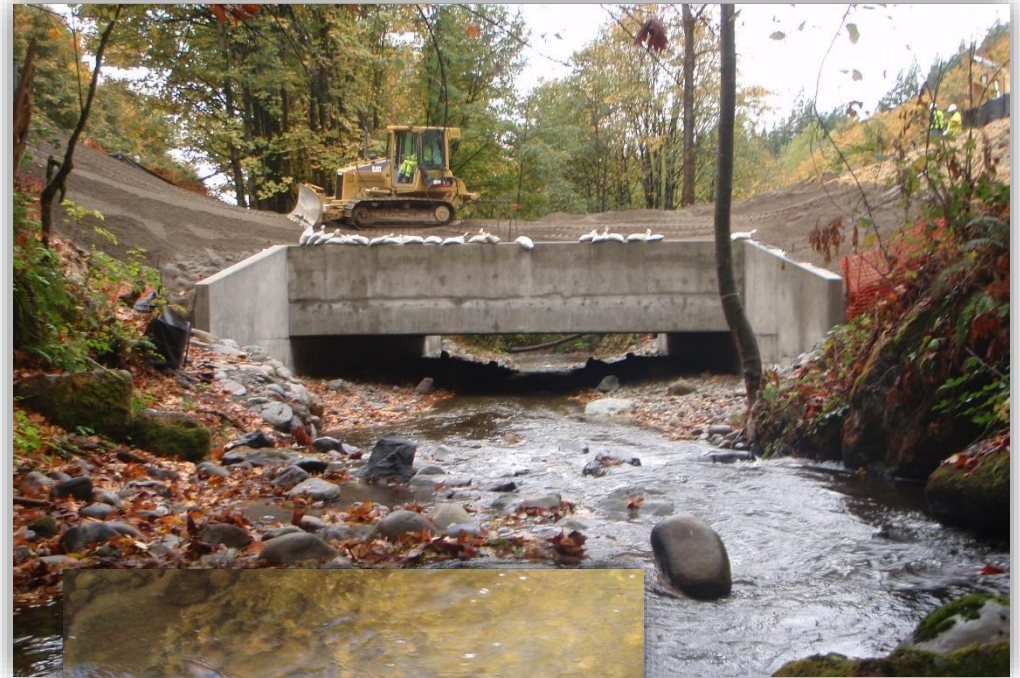
After - 26 Foot Bridge
