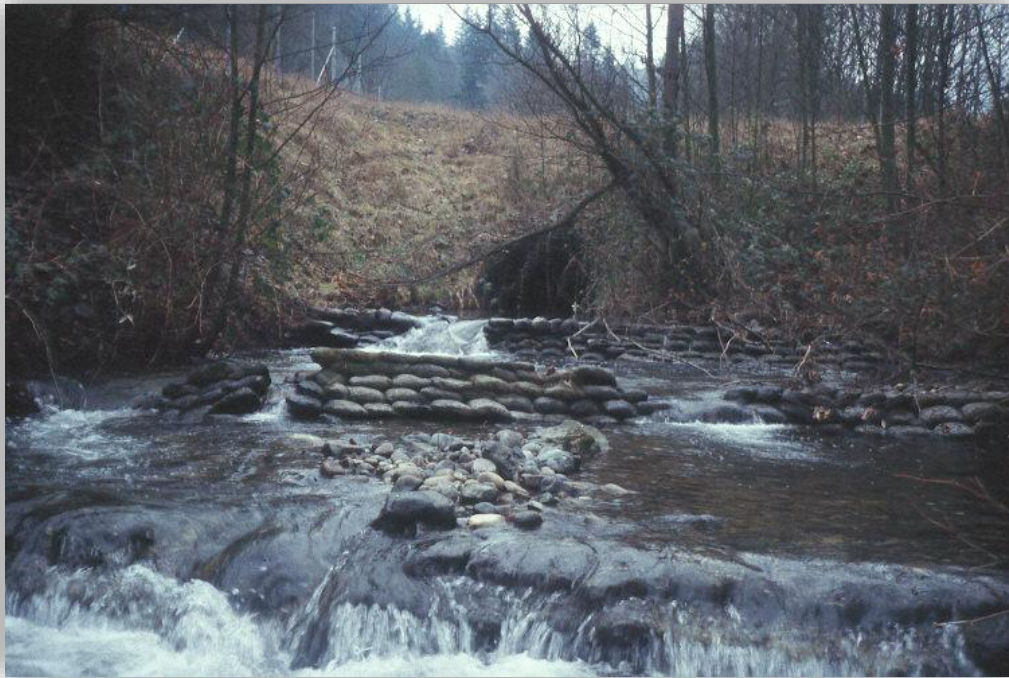
Before – 12 Foot Culvert
