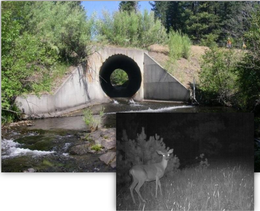
Before – 10.5 Foot Culvert
