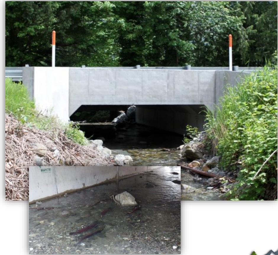
After - 17 Foot 3-Sided Structure
