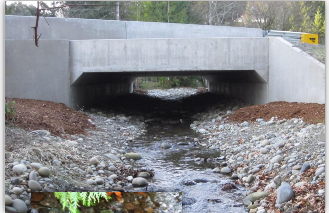
After - 20 Foot 3-Side Structure
