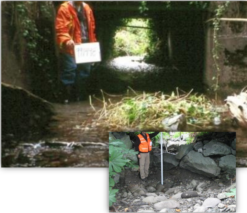
Before – 8 Foot Culvert
