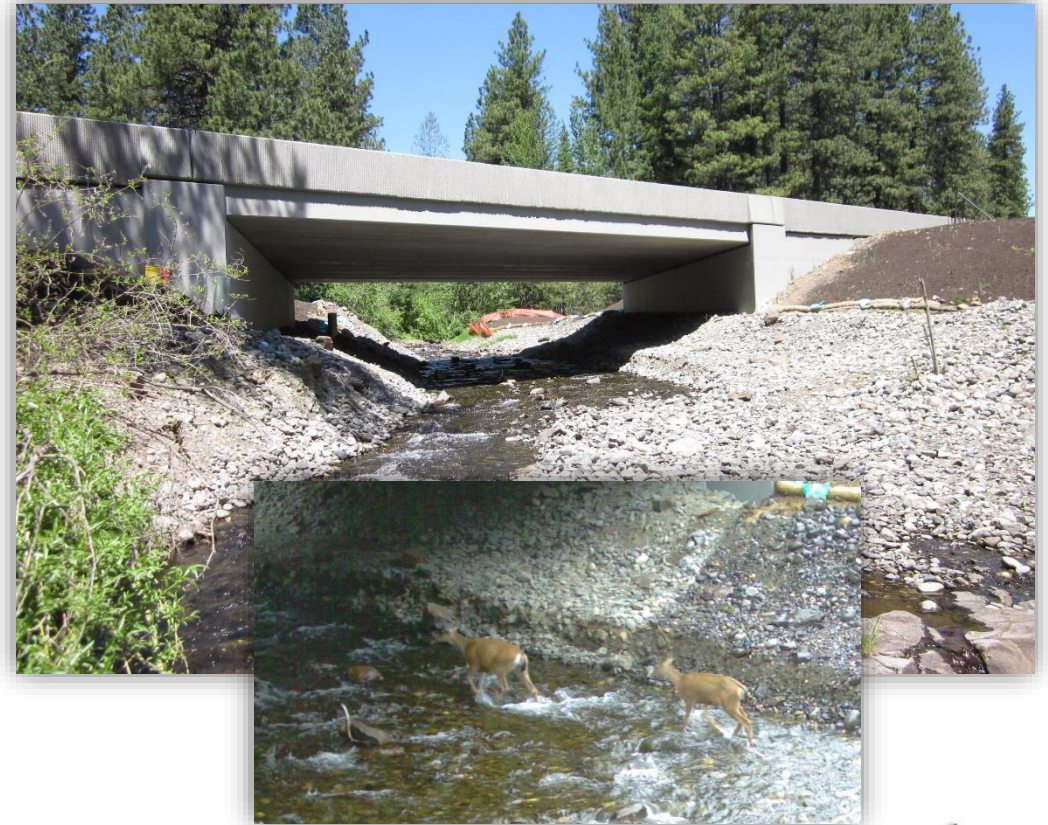
After - 65 Foot Bridge
