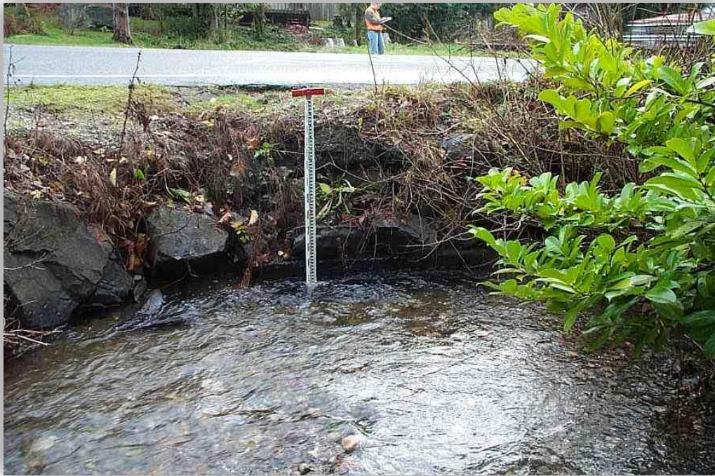
Before - 4 Foot Box Culvert
