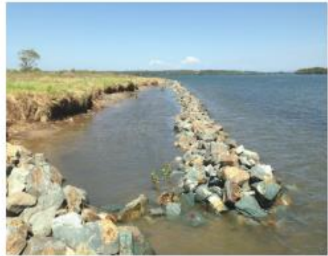
Newly installed rock fillet, rock fillet protecting saltmarsh, mangrove trees behind rock fillet
