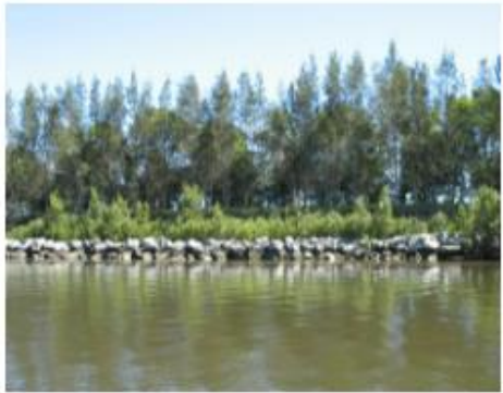
Newly installed rock fillet, rock fillet protecting saltmarsh, mangrove trees behind rock fillet
