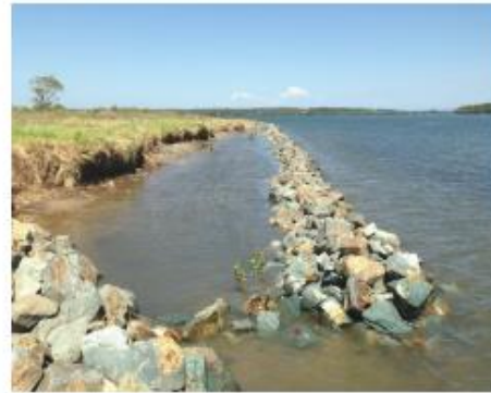
Newly installed rock fillet, rock fillet protecting saltmarsh, mangrove trees behind rock fillet
