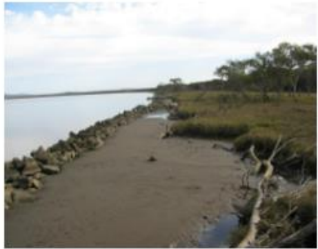
Newly installed rock fillet, rock fillet protecting saltmarsh, mangrove trees behind rock fillet
