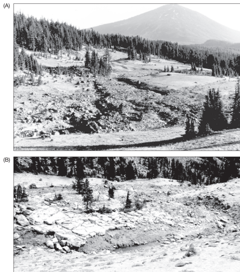
Fig. 16 Areas of erosion and deposition from Oct. 7, 1966, moraine-dammed-lake outburst at terminus of East Bend Glacier at Broken Top volcano, central Oregon Cascade Range, United States. (A) Downstream view of fan of 1–2 m boulders deposited about 2.1 km downstream of breach. (B) Evident erosion, probably by plucking and toppling, of jointed basaltic andesite flows along the valley bottom, about 1.6 km downstream from the breach; flow left to right. Modified from O'Connor JE, Hardison III JH, Costa JE (2001) Debris Flows From Failures of Neoglacial Moraine Dams in the Three Sisters and Mt. Jefferson Wilderness Areas, Oregon. U.S. Geological Survey Professional Paper 1608, 93pp.
